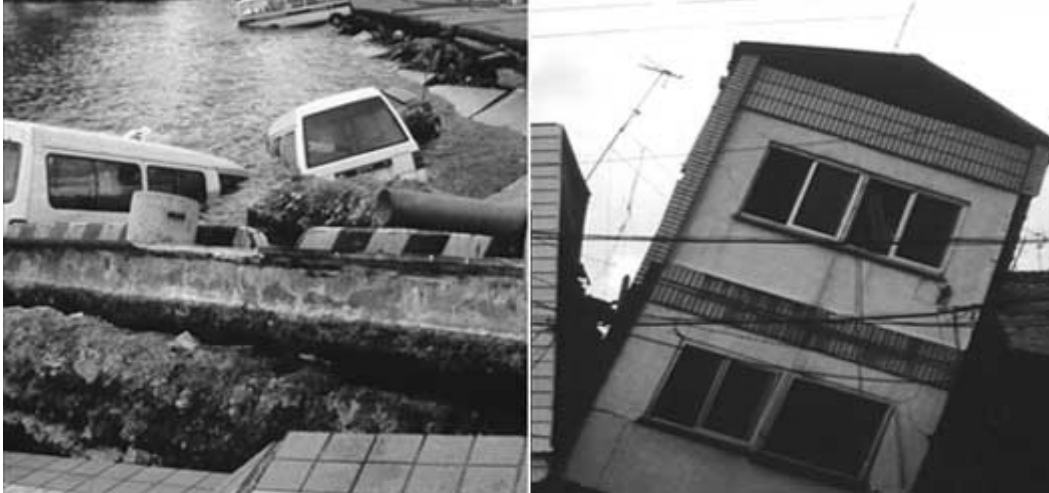
Aftermath of the Kobe earthquake of 1995. It measured 6.9 on the Richter scale.
